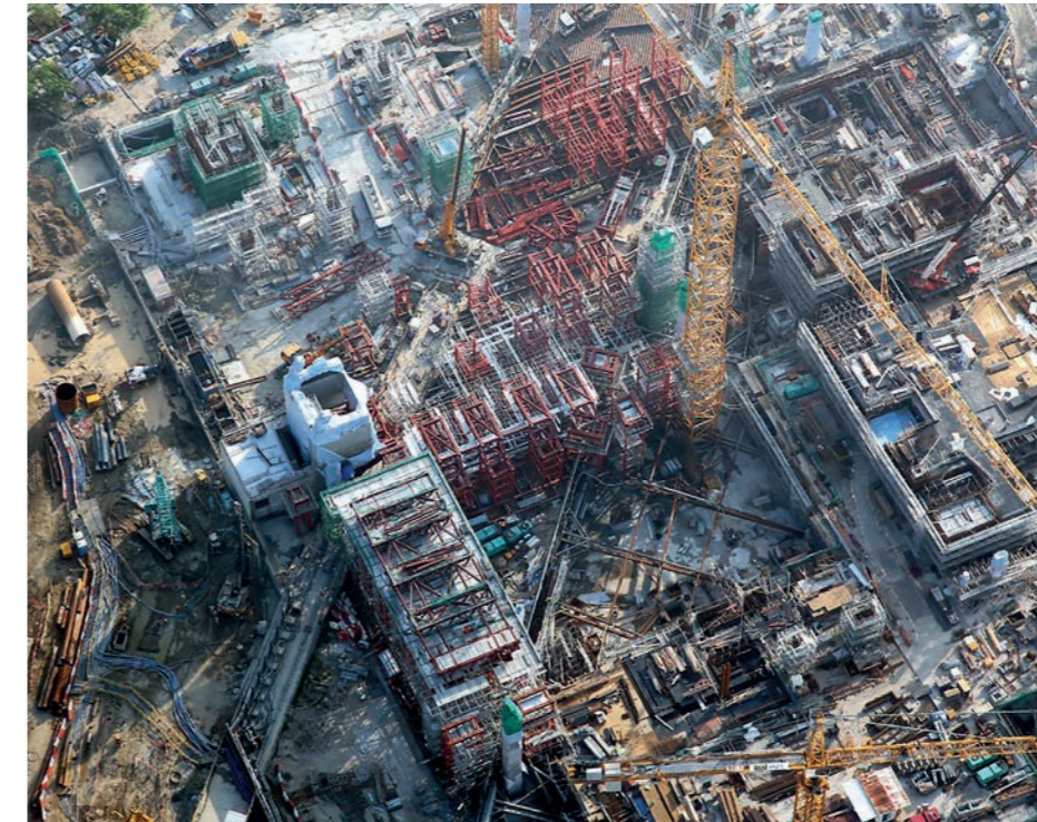
Aerial view of M+ Museum Hong Kong under construction
