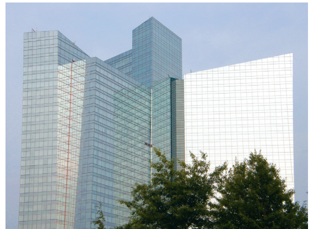
Fig. 1.1 Casino: Completed in 2001, Connecticut's Mohegan Sun Casino is an early example of a full virtual modelling project (today known as BIM)
