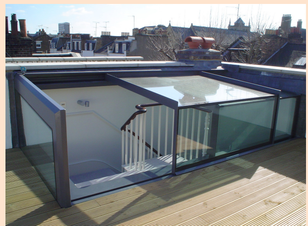
Fig. C8 Box Rooflight Installed
